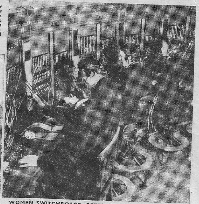
WOMEN SWITCHBOARD OPERATORS at the London Region Fire Control Room, headquarters of the N.F.S. This switchboard is the nerve centre through which the operations officer receives reports of fires and through which he issues his fire-fighting orders.
