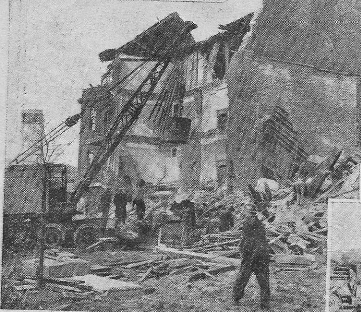
CIVIL DEFENCE PERSONNEL labour doggedly, with a mobile crane, to clear away debris after a direct hit. Folks may be trapped beneath the rubble masses: men of the Rescue Service attend to these when contact has been made.
